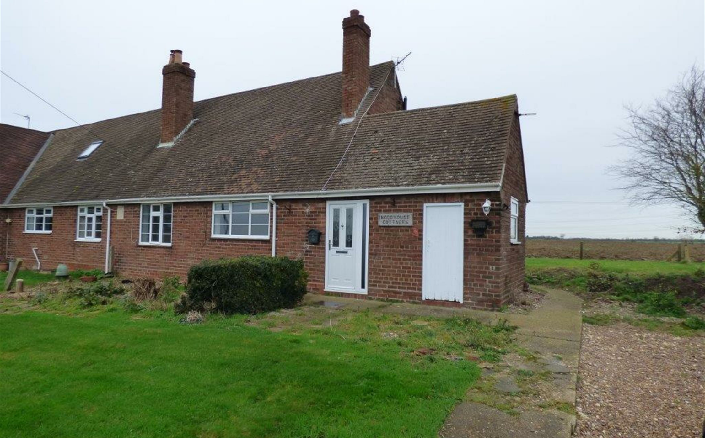
1 Woodhouse Cottages Swine, East Yorkshire, HU11 4JH
