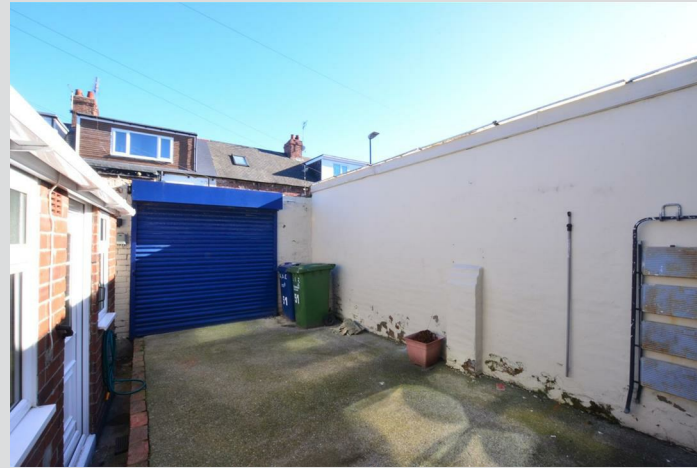
Rear courtyard, with a remote controlled roller shutter garage door.
