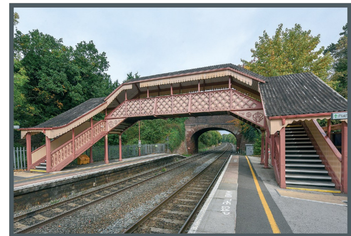
Hagley Train Station
