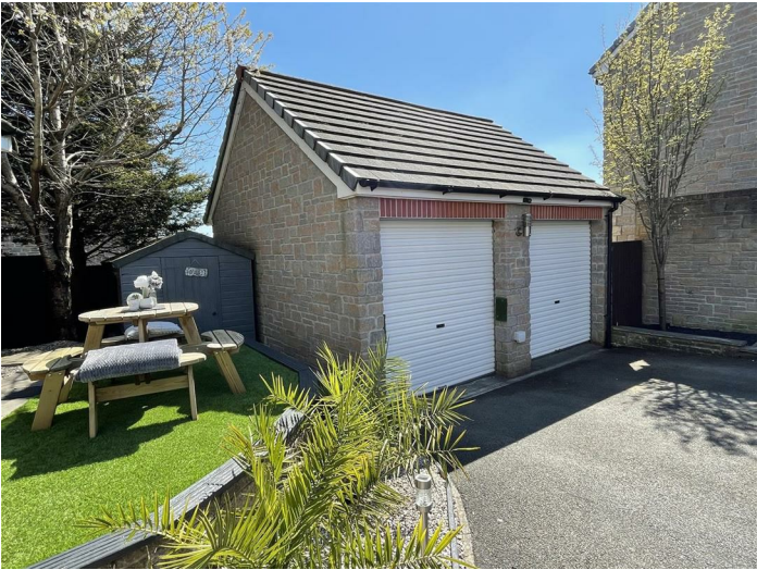
Twin up and over garage doors. The garage benefits from light, power and eaves storage. A fantastic space.
