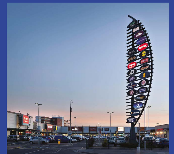
Tottenham Retail Park tottenhamhaleshopping.co.uk
