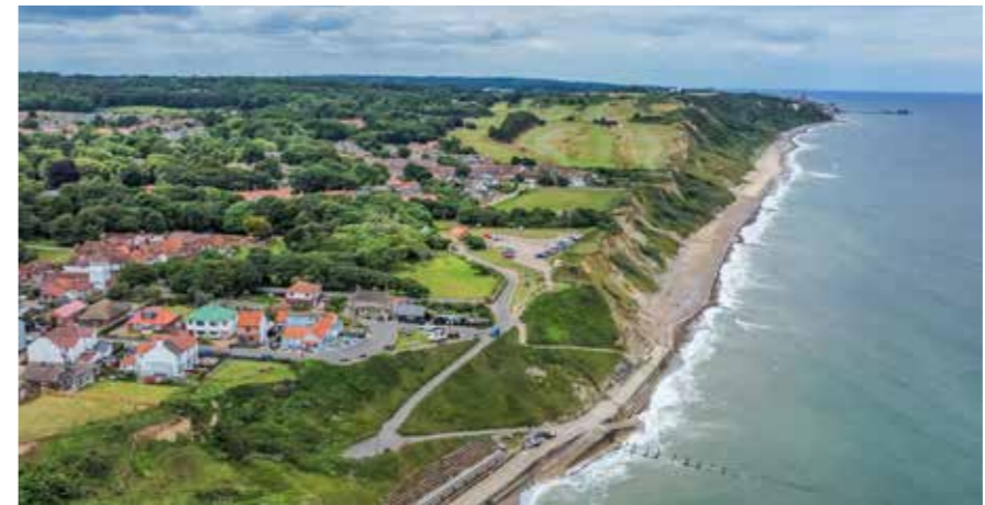
29 Cliff Road and its surroundings.
