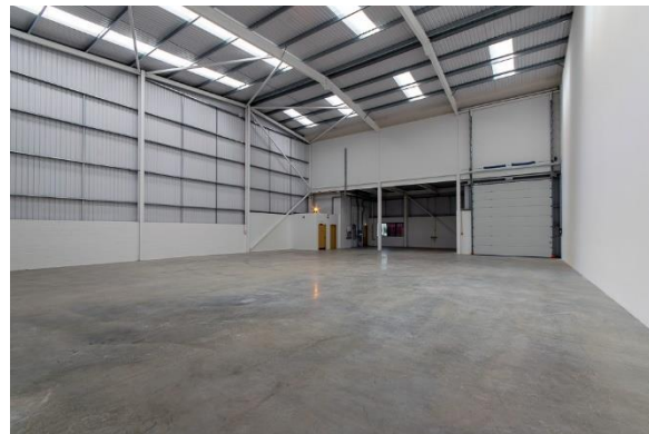
Photo showing typical example of warehouse on the Estate
