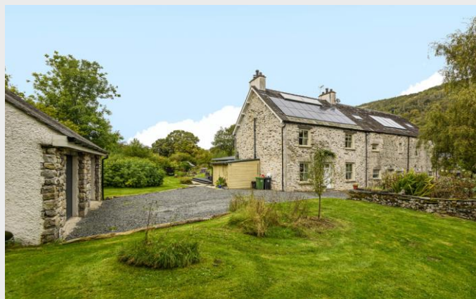
House, Grounds & Garden
