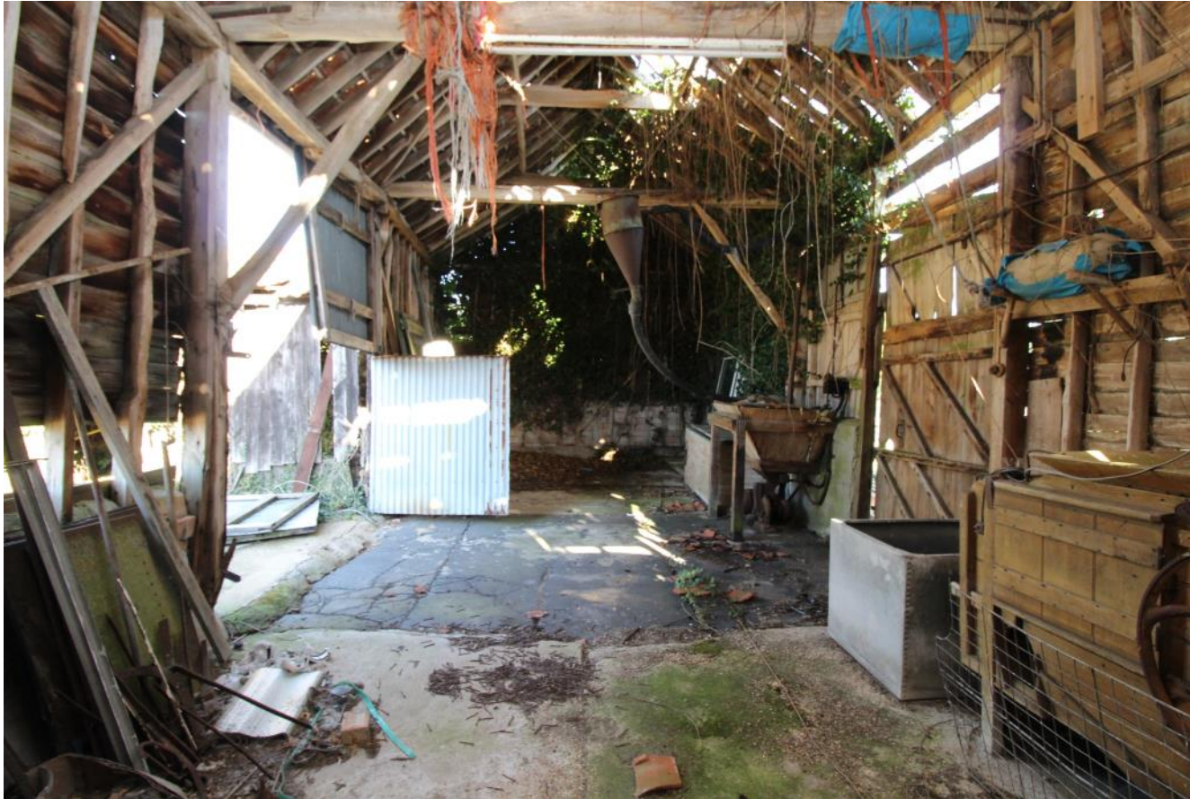
Wood Farm Barns - Main barn
