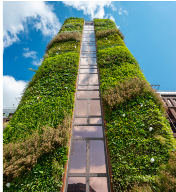
▲ Exterior living 'green' wall
