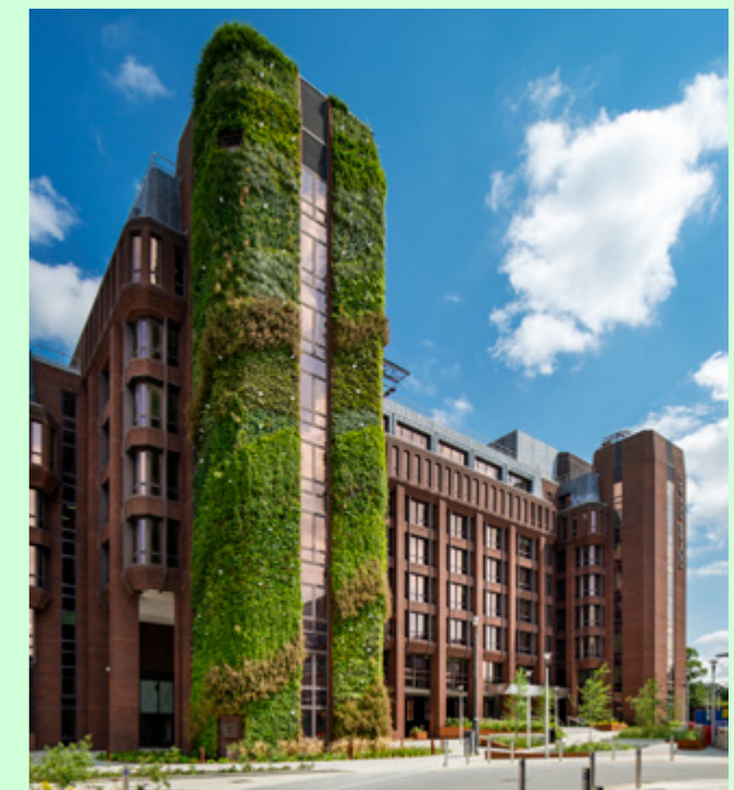
▲ Exterior living 'green' wall
