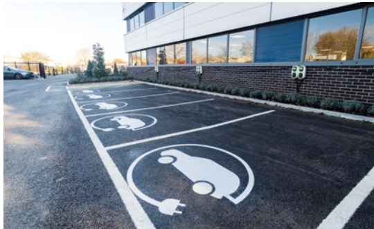
Westerly elevation showing electric vehicle charging points
