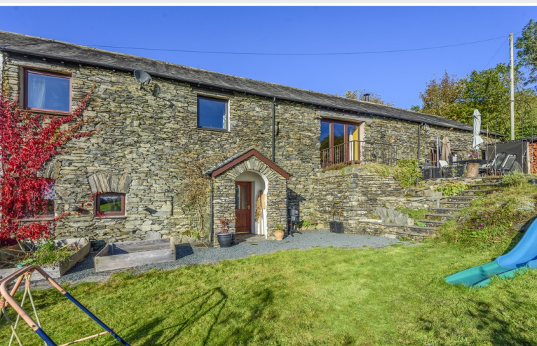
Front of Property
