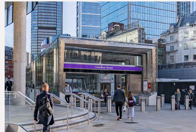
Top Liverpool Street station upper escalator with inclined lift to Broadgate ticket hall Bottom Liverpool Street station entrance at Broadgate
