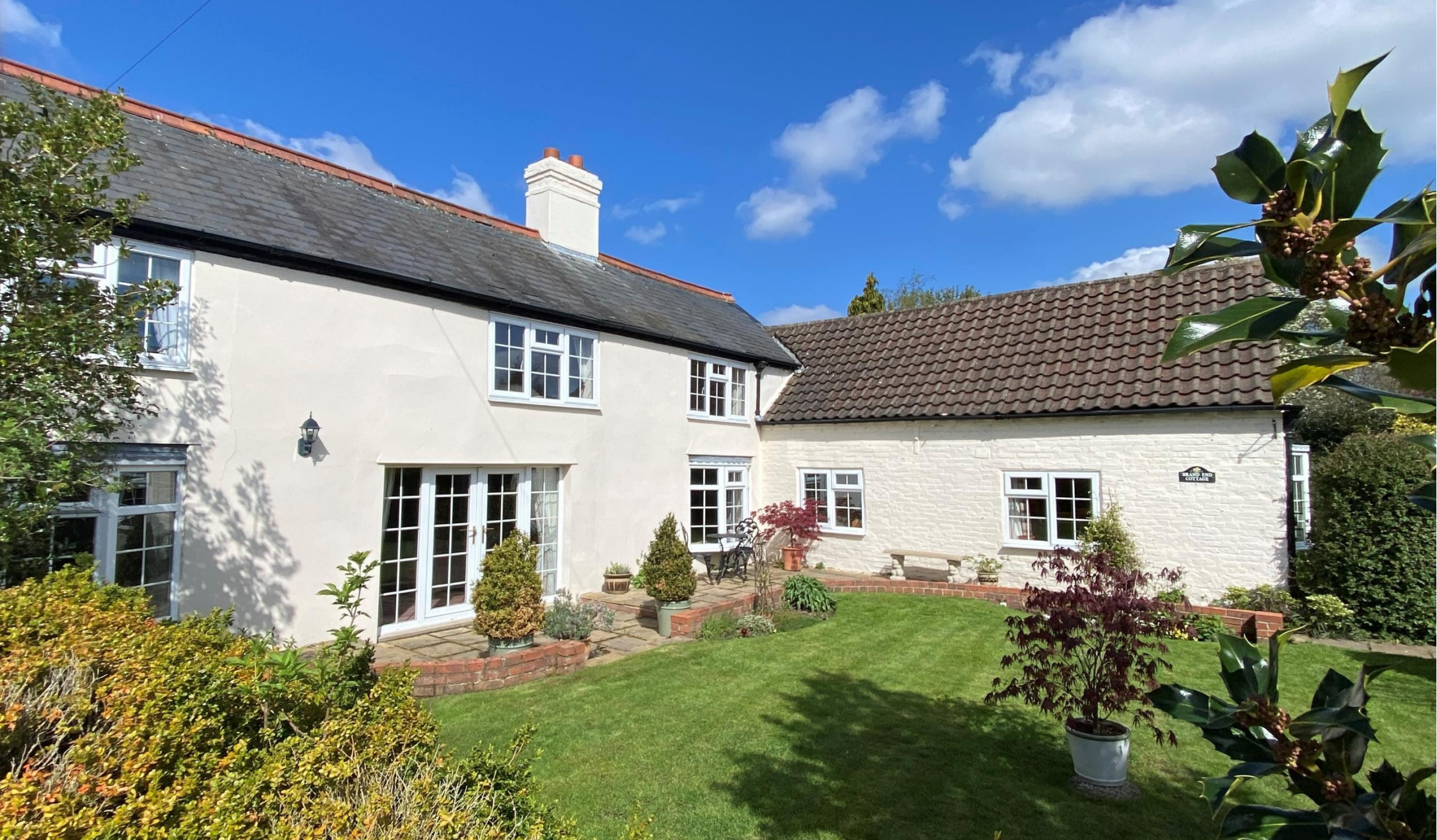
BRAND END COTTAGE, 29 RECTORY LANE, GAMSTON £425,000
