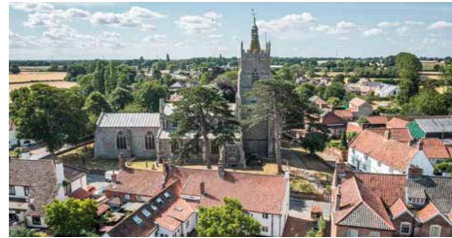
View of the Church from behind the row of properties opposite.
