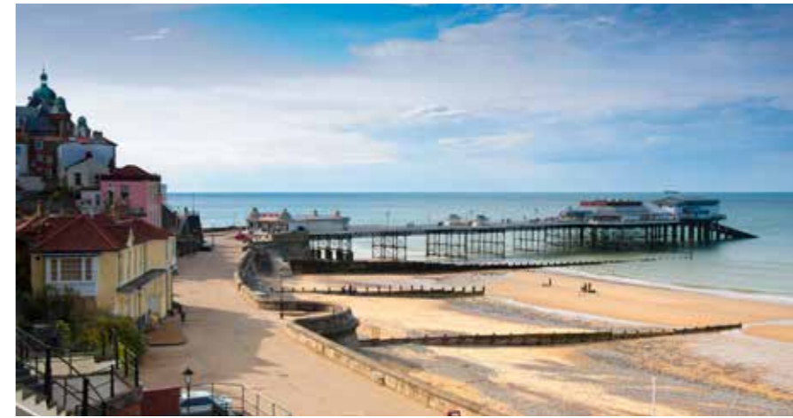
Cromer Pier and seafront.
