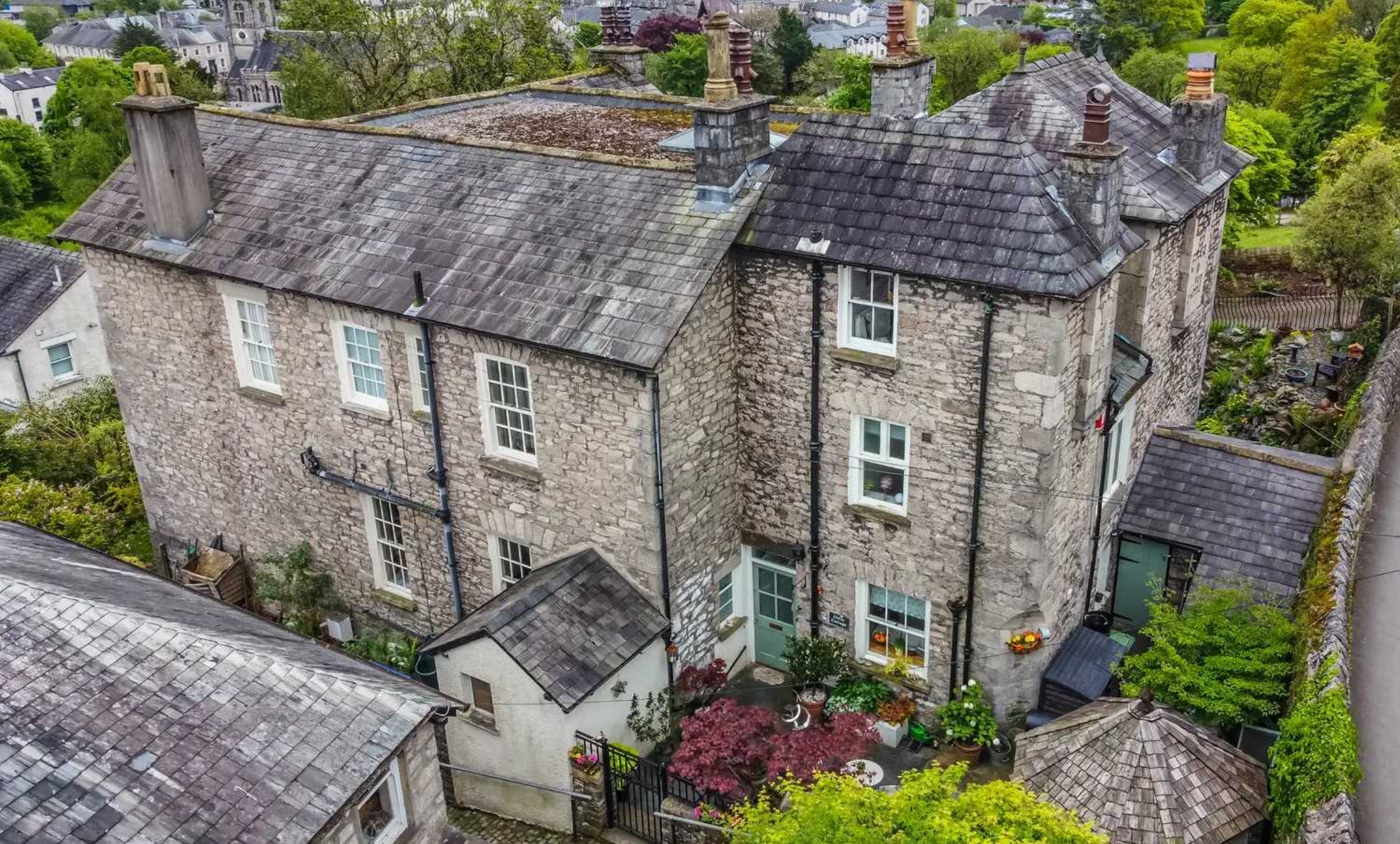
Glebe Cottage Queens Road, Kendal £350,000
