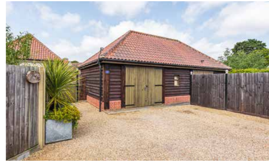
The garage/workshop at 2 Old Stables.
