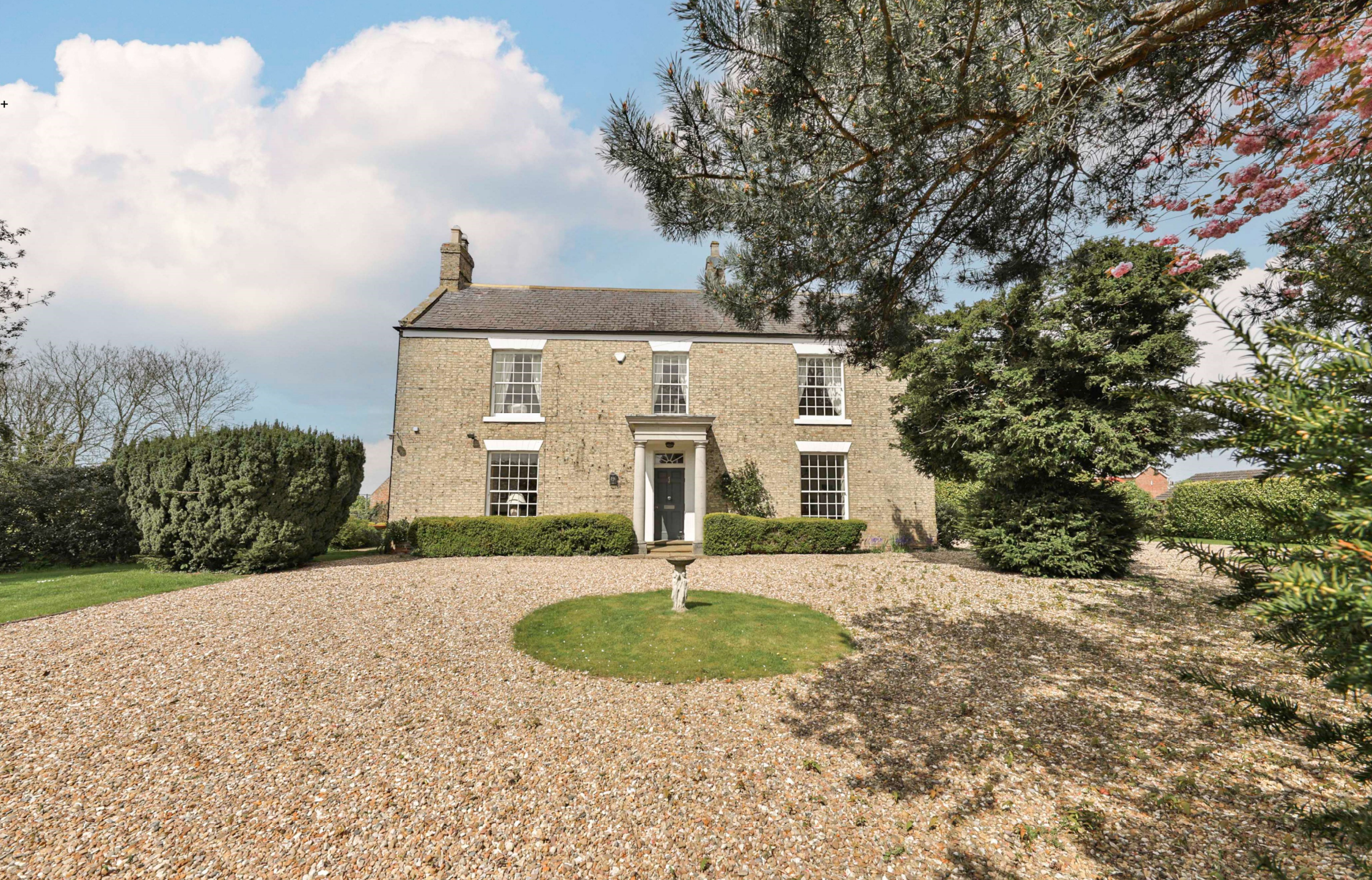
Back Lane, Burstwick, East Riding of Yorkshire
