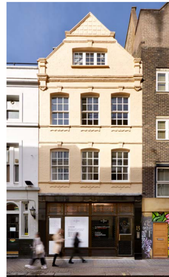
In the restored facade, classic Soho architecture is alive and well.
