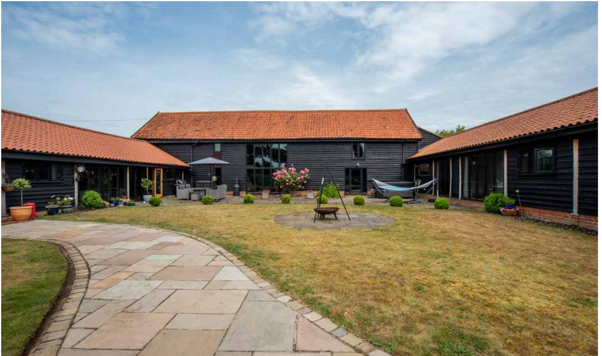
Manor Farm Barn Fressingfield Road | Stradbroke | Suffolk | IP21 5NJ
