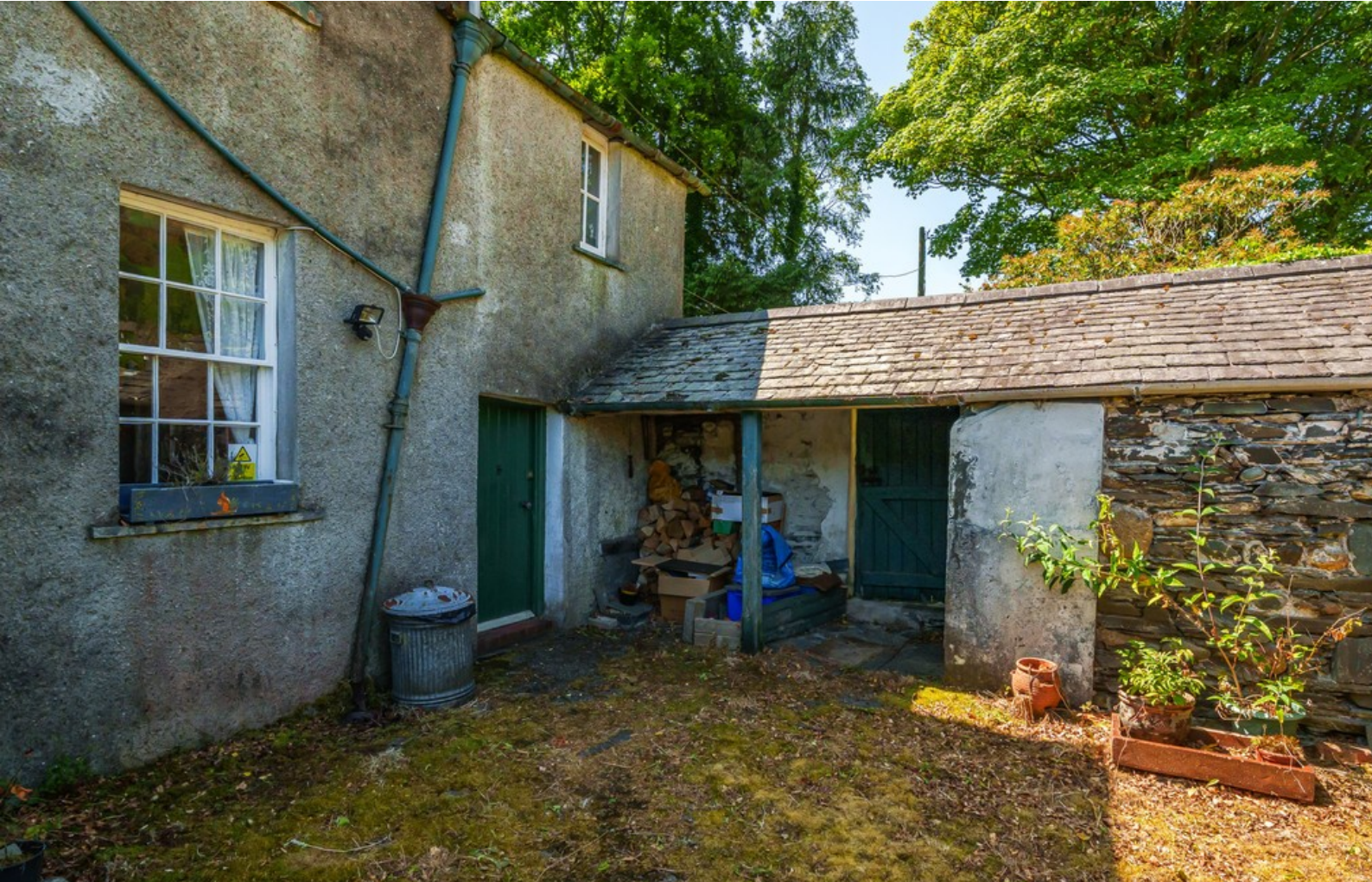
Open Stores and Rear Yard
