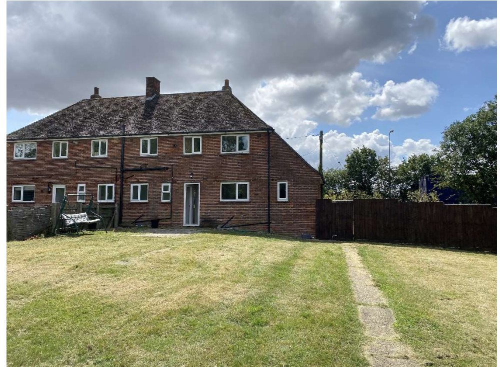
Rear of house
