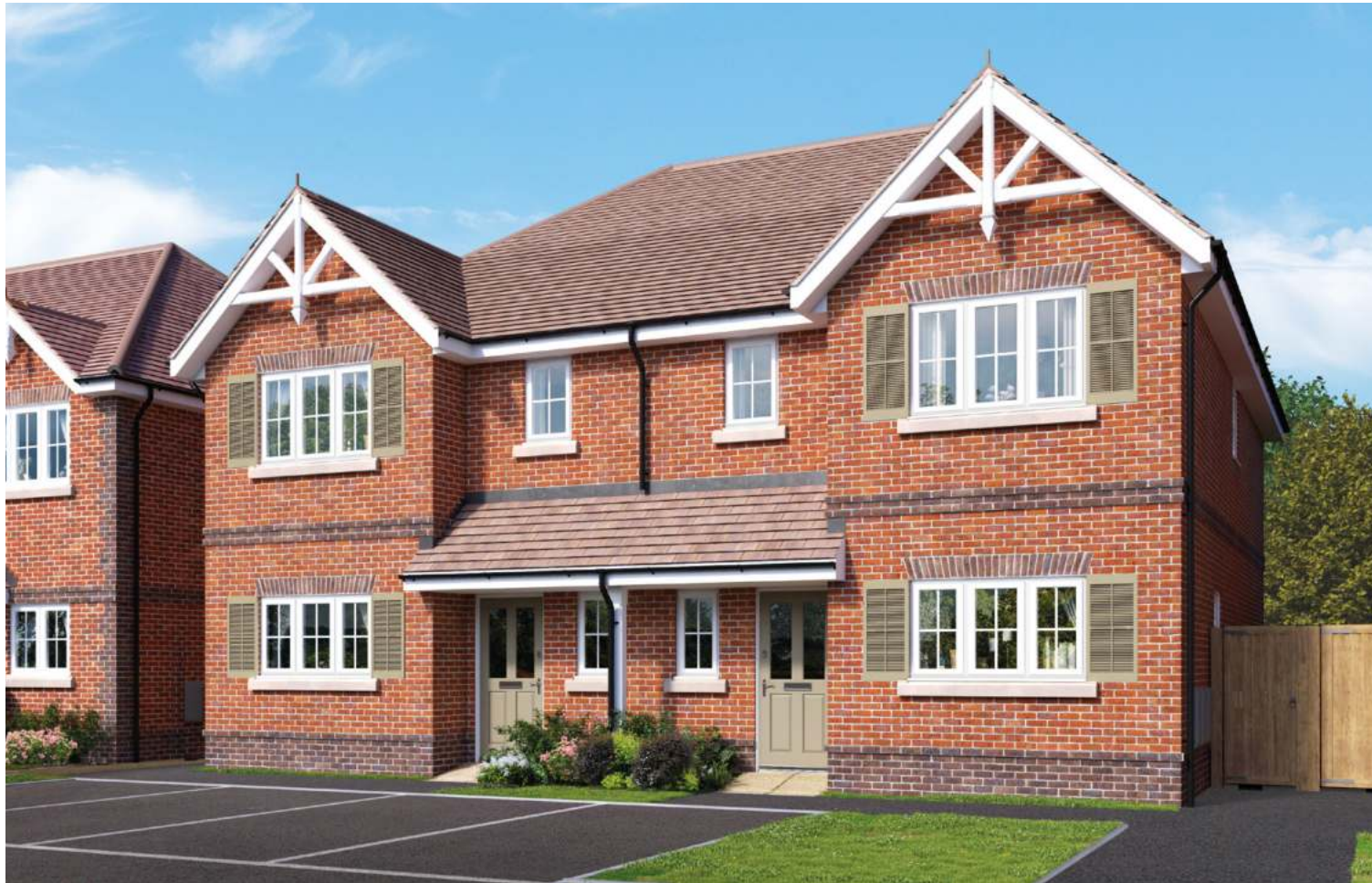
Computer generated imagery of Plots 8 & 9 indicative only. Please note, elevations may vary. Shutter colours may vary.
