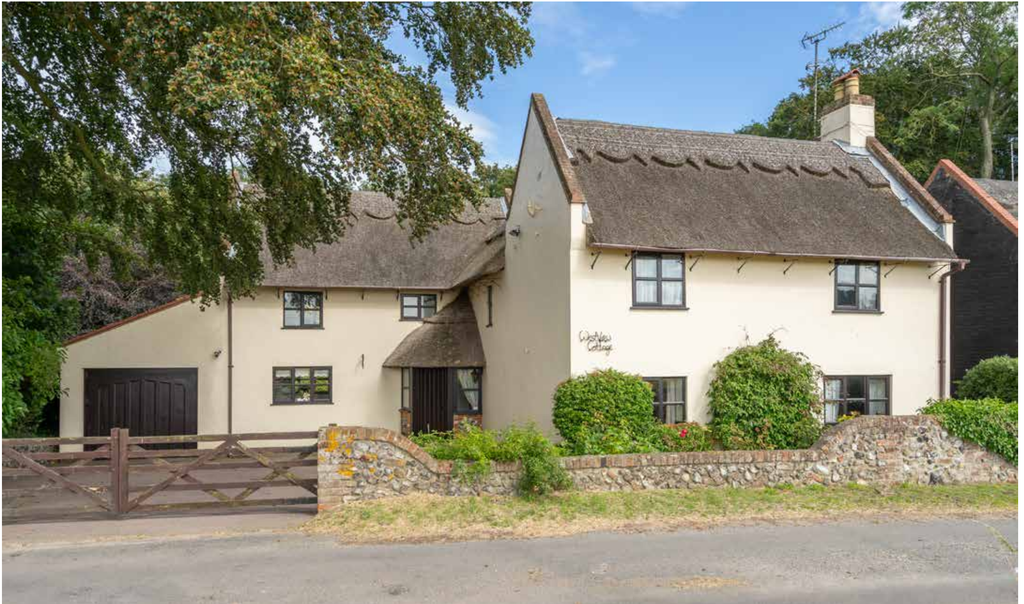
West View Cottage Sandy Lane | West Somerton | Norfolk | NR29 4DJ
