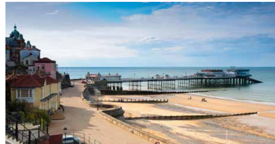
Cromer pier and seafront
