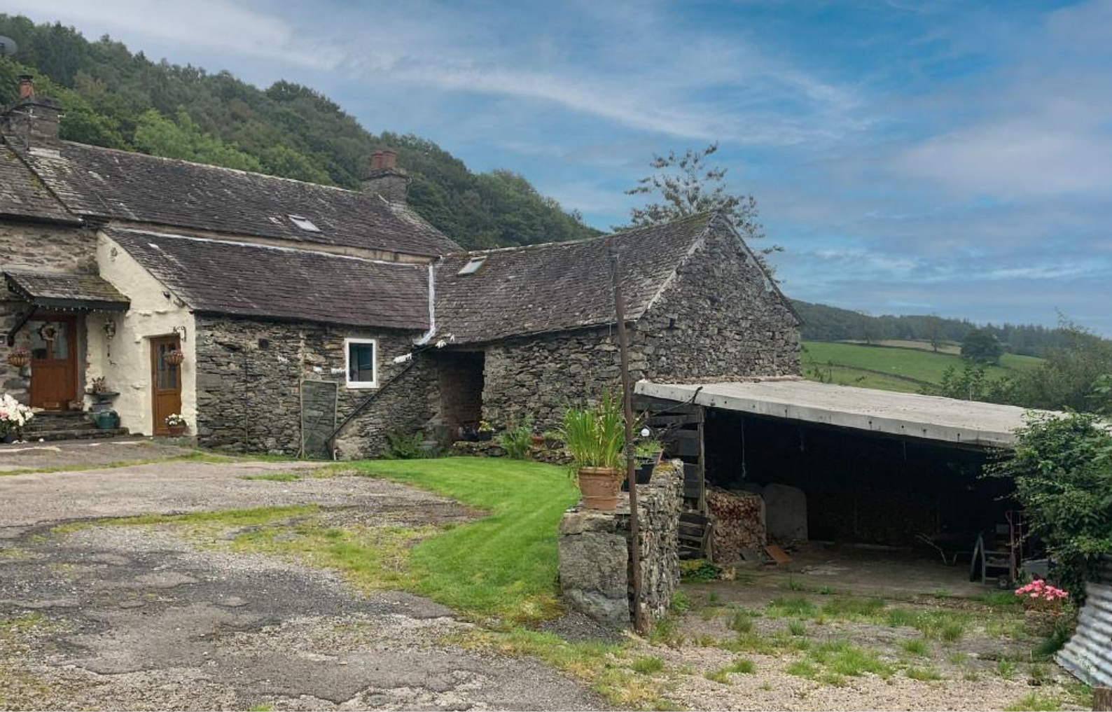
RearAspect, Barn and Double Garage
