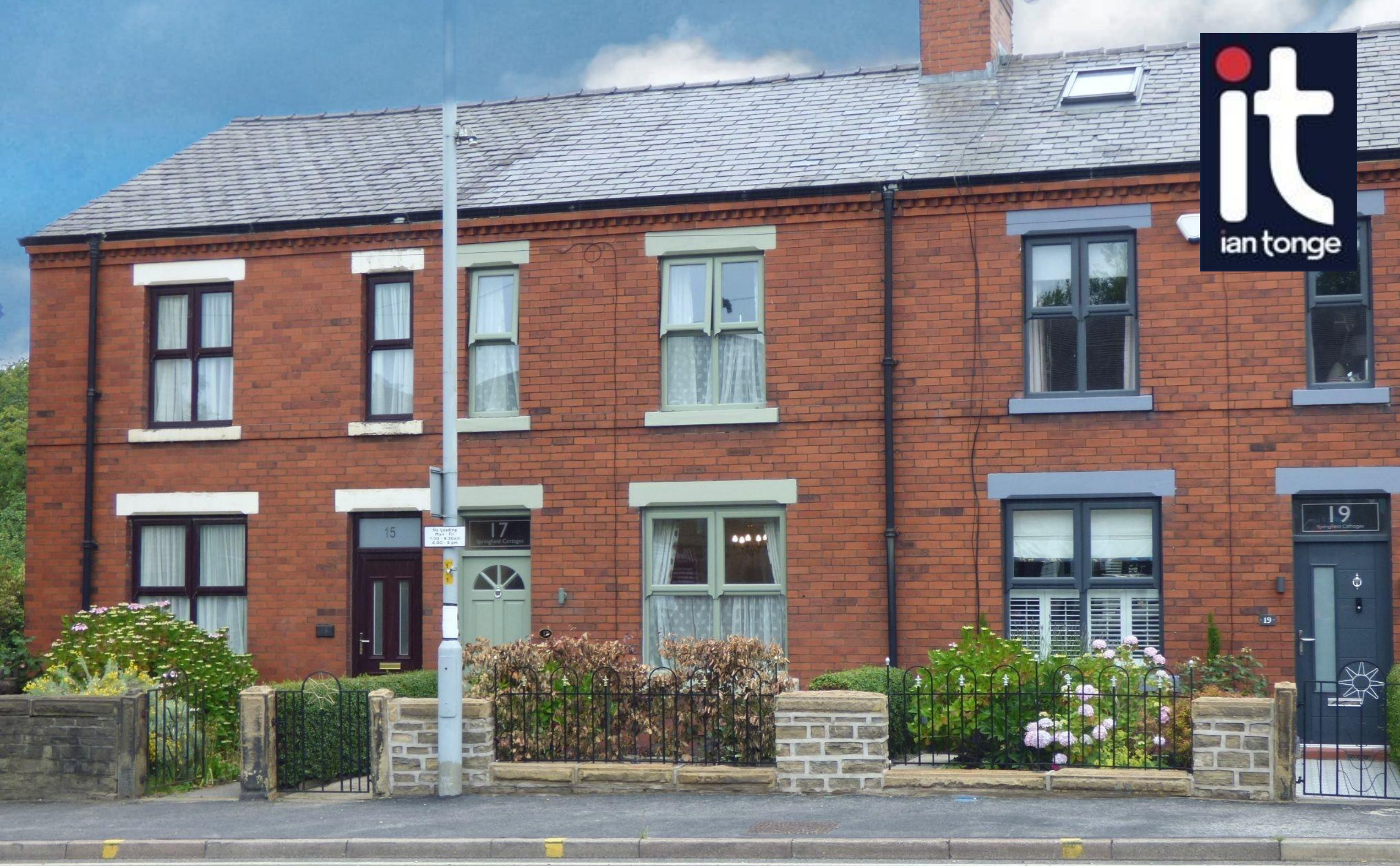
Springfield Cottages, Buxton Road, High Lane, SK6
