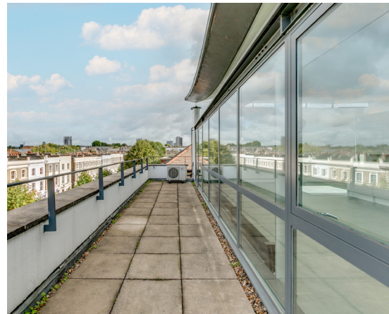
4th floor terrace
