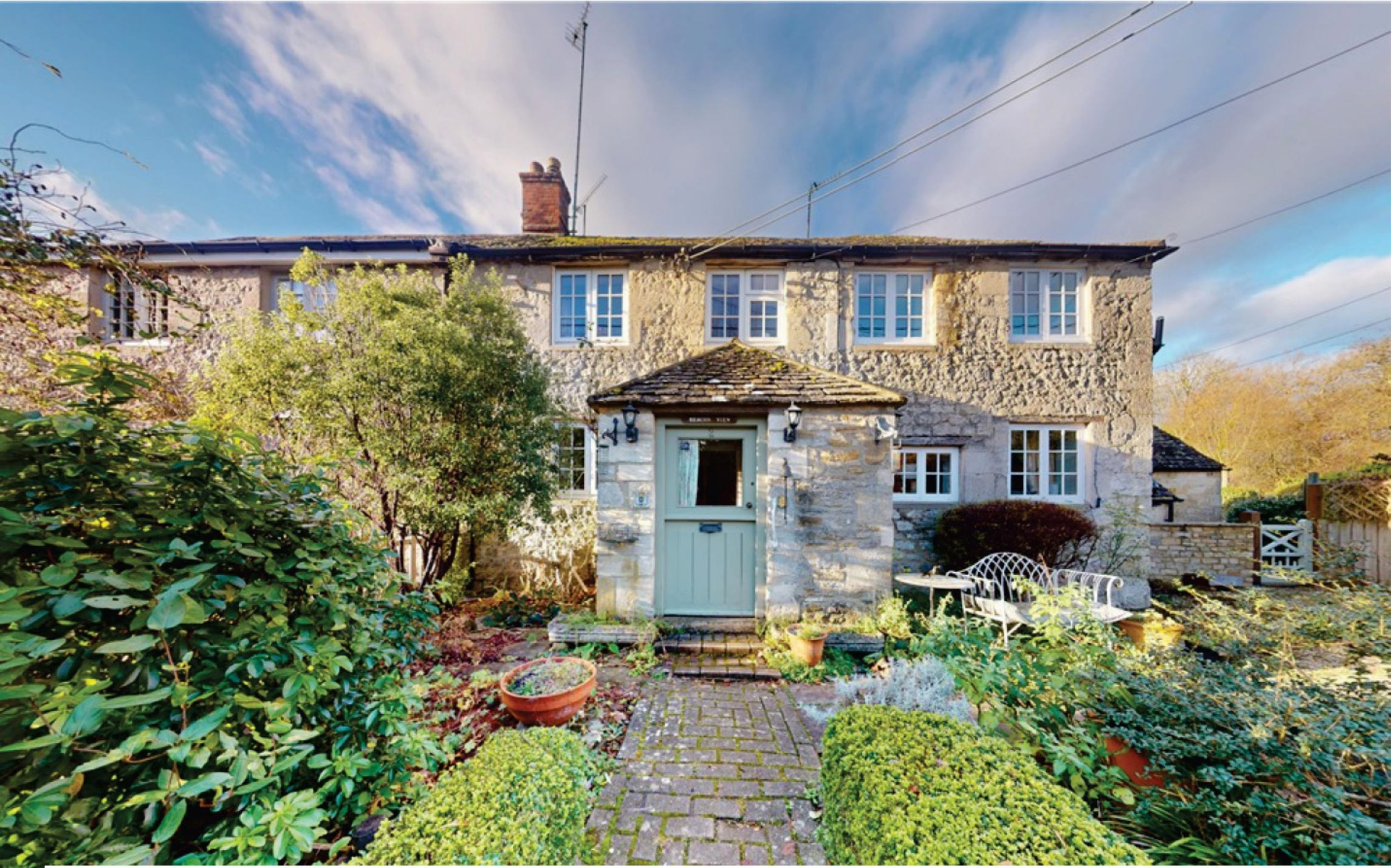
Beacon View, Swinford
