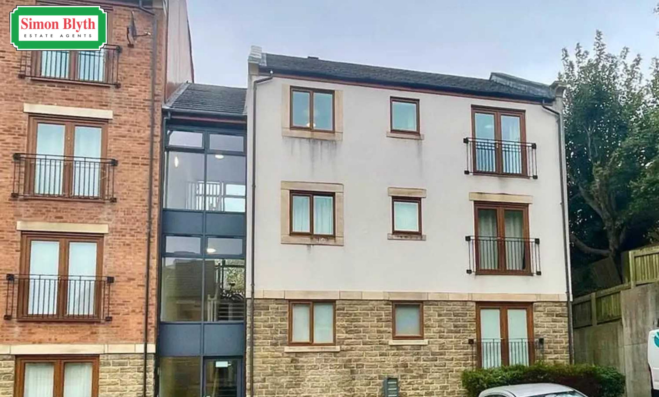
180 Greenlea Court, Huddersfield Huddersfield
