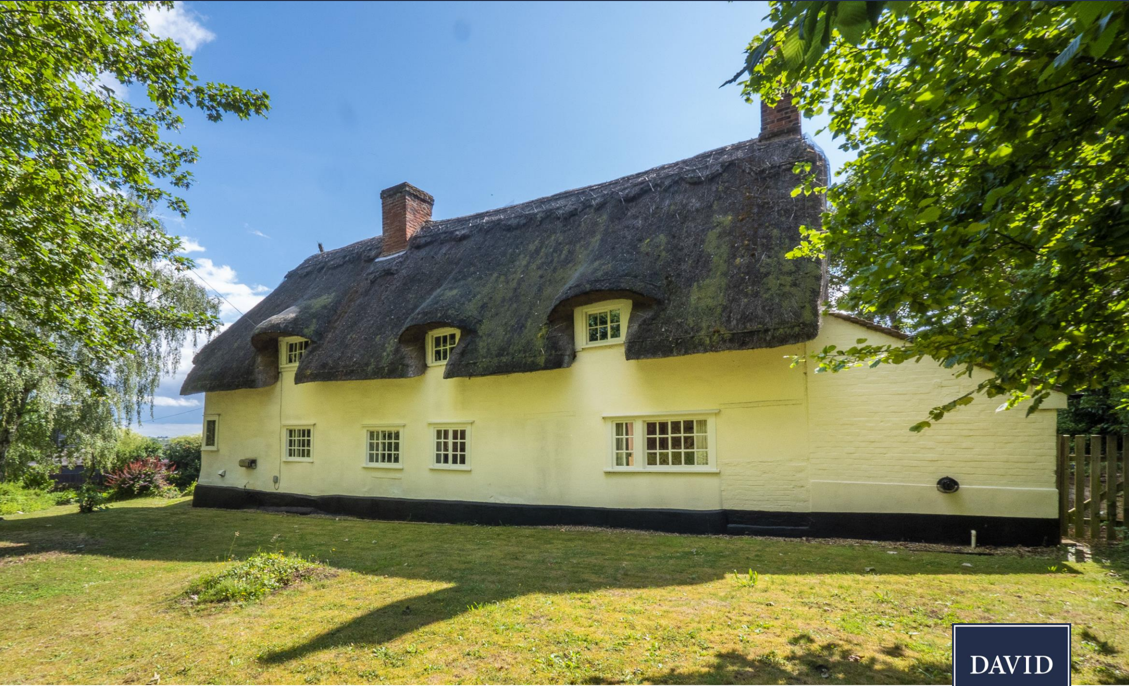
Allens Cottage Sudbury Road, Bures, Suffolk
