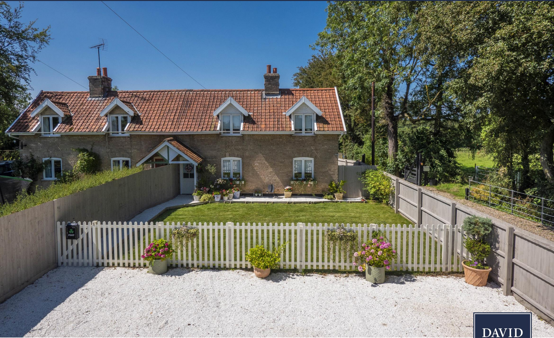
1 Jaggards Cottage, Thorpe Morieux, Suffolk
