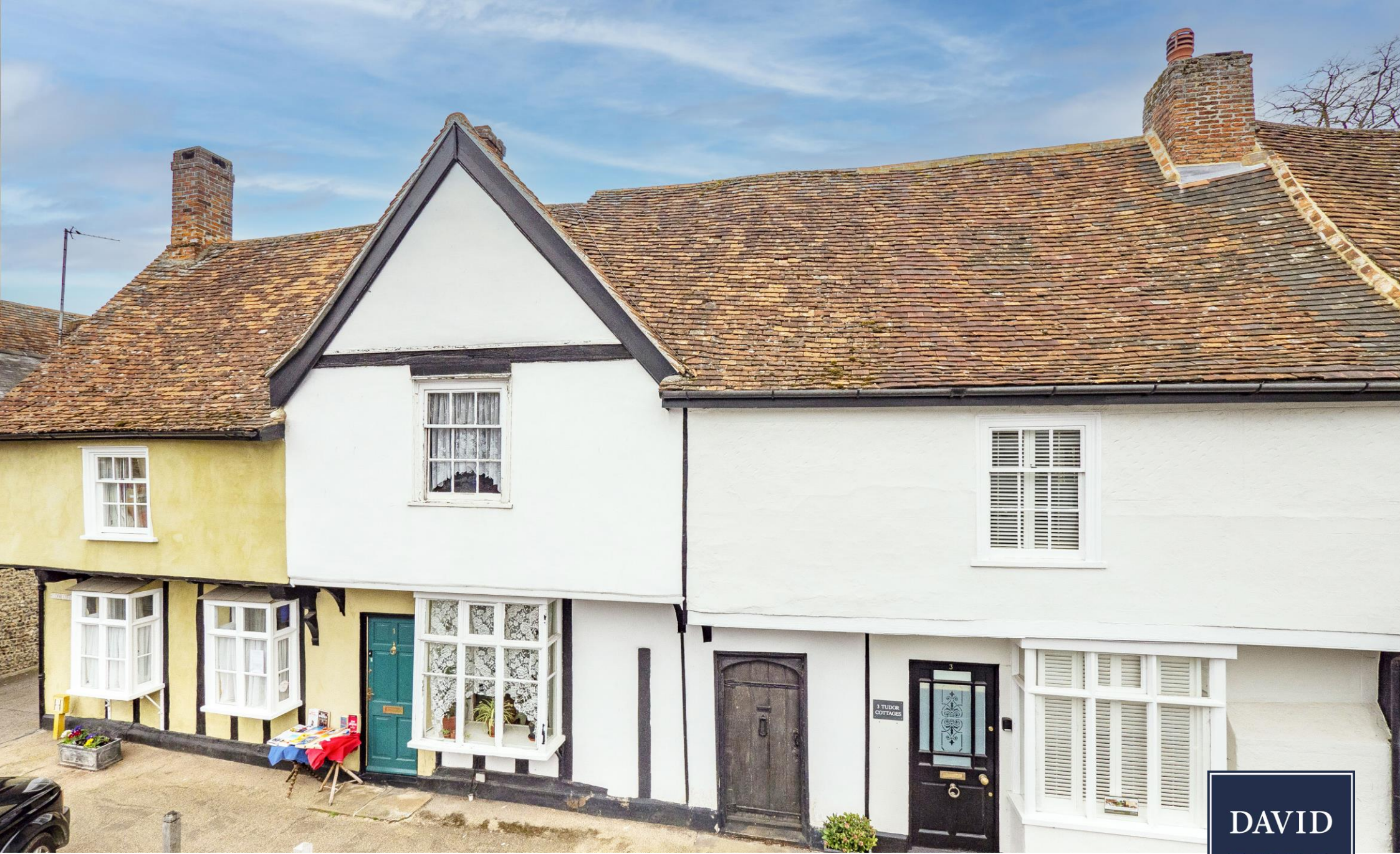
2 Tudor Cottage, Hall Street, Long Melford, Suffolk
