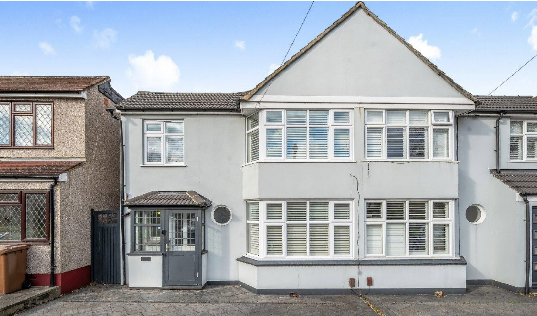
Willersley Avenue, Sidcup, DA15 Approximate Area = 1213 sq ft / 112.6 sq m For identification only - Not to scale
