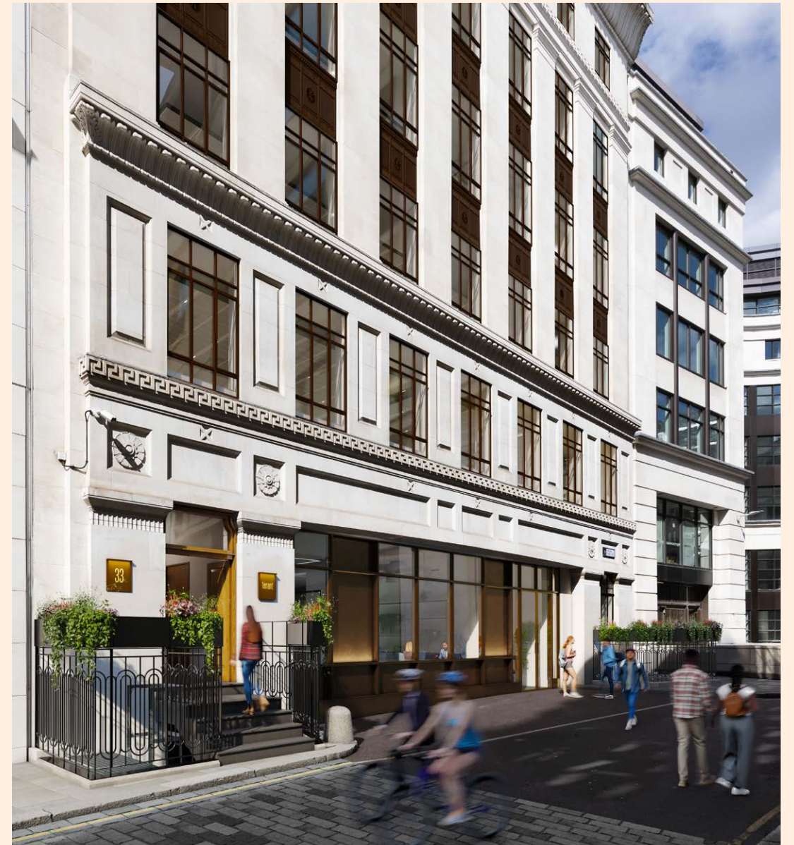
View of the rear Foster Lane entrance
