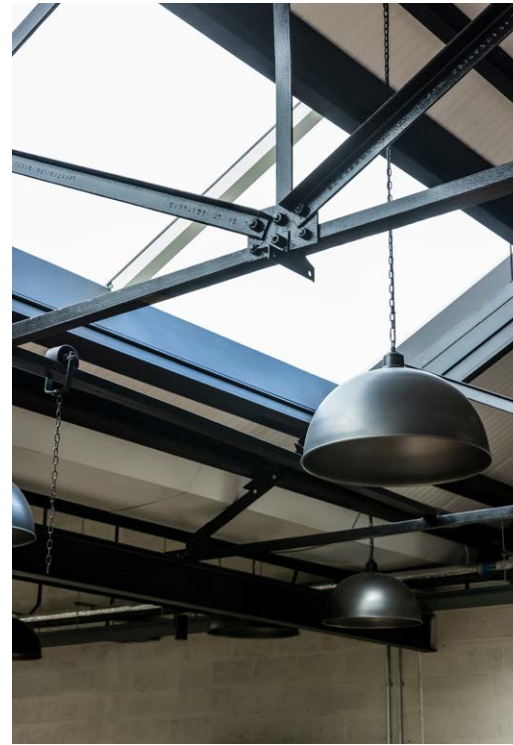
Refurbished Steel Beams
