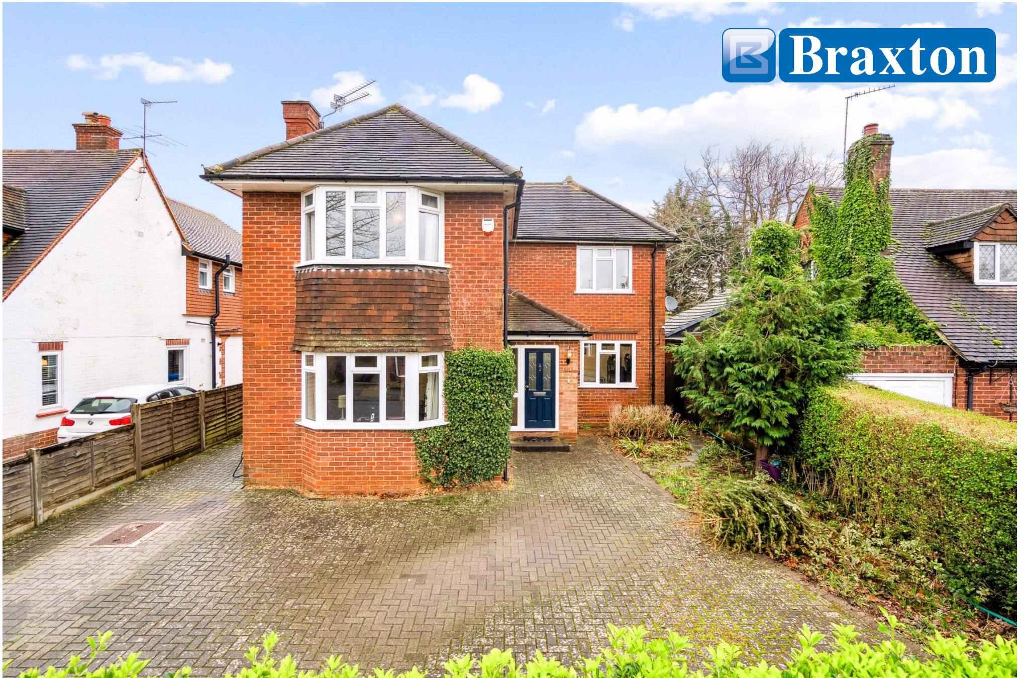
62 Oaken Grove, Maidenhead, Berkshire SL6 6HH
