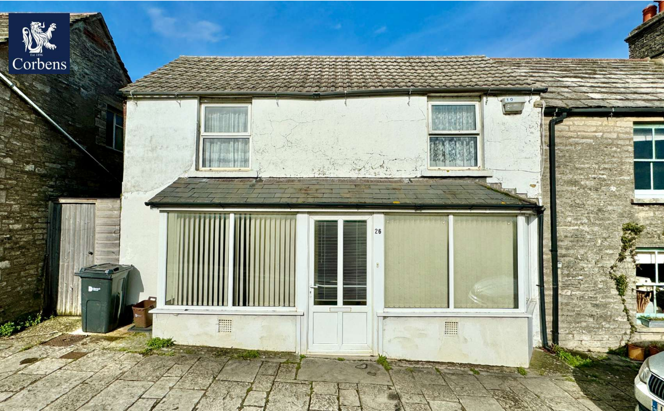
26 HIGH STREET, LANGTON MATRAVERS £445,000
