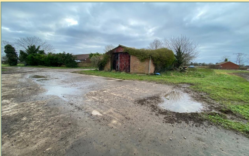
BUILDINGS TO BE DEMOLISHED
