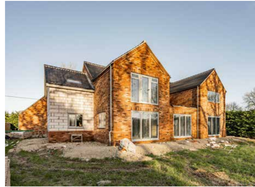
Build Progress as of January 2024.
