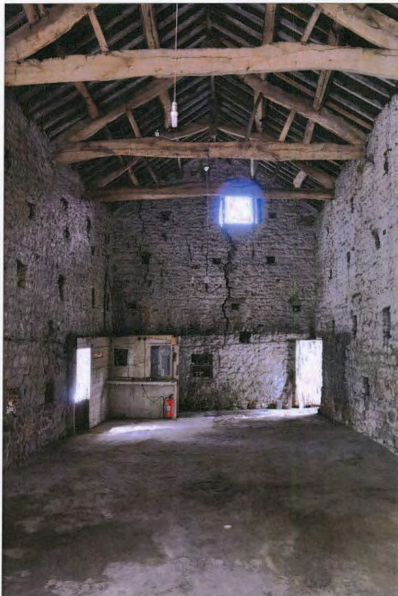
Photo 7: Interior: north-west end
