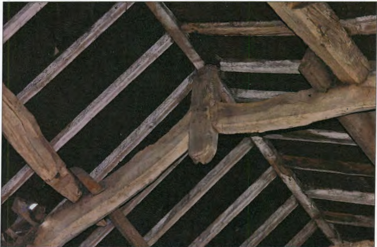
Photo 6: King-block truss, over north-west end of barn
