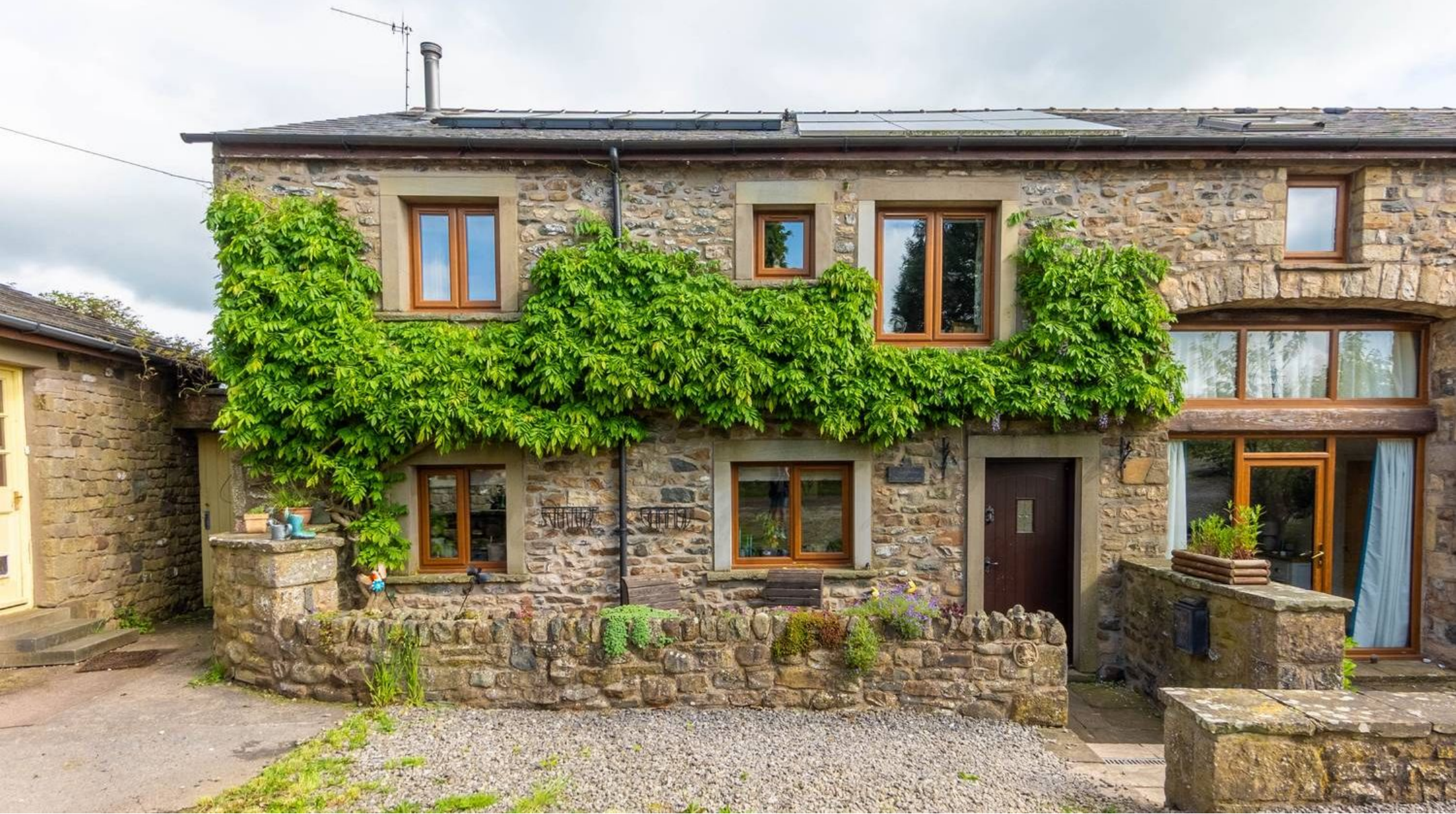
Collingholme Barn Cottage, Cowan Bridge £600,000 Freehold
