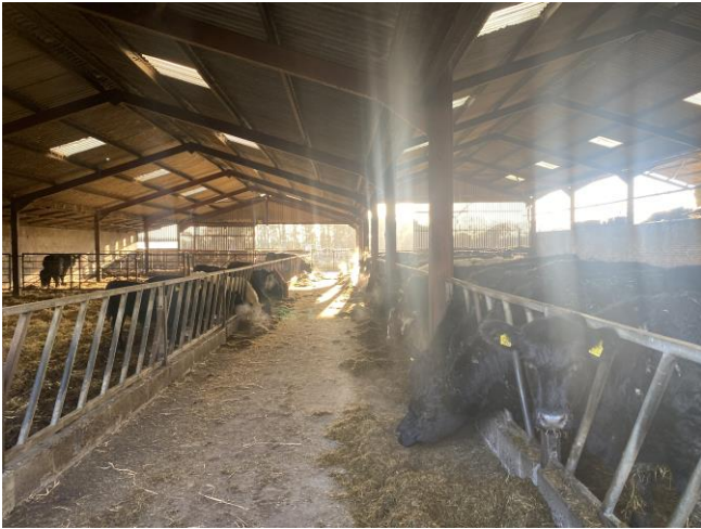
Covered Silage Pit: – 45'9" x 118'11" Steel framed with concrete panel walls, corrugated asbestos roof, box profile sheeted side cladding and concrete floor.
