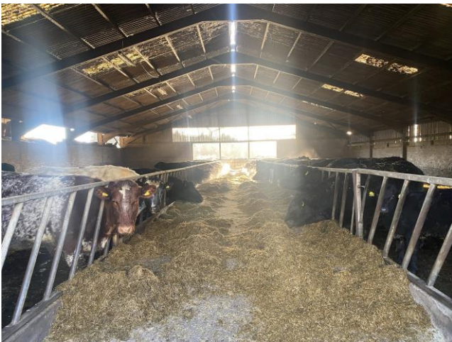
Tup Shed: 21'3" x 12'1" Timber framed, corrugated iron roof and sides.
