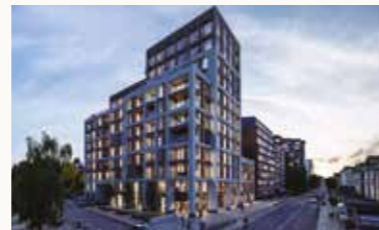
CARLTON HOUSE, LONDON SW15
