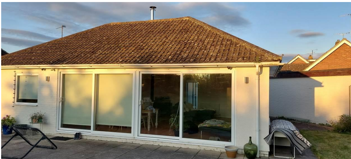
Photo A3: Dwelling and hardstanding
