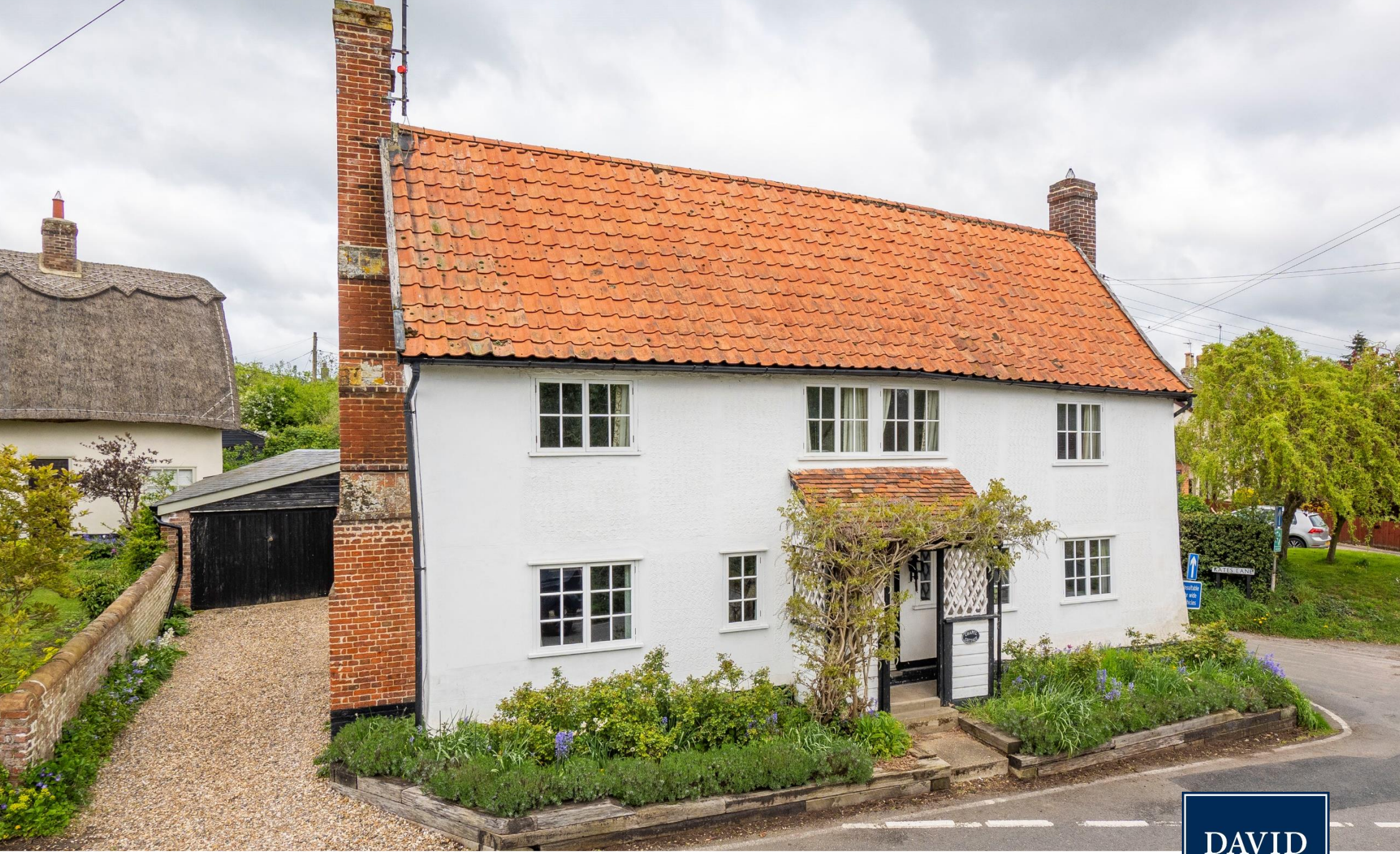
Chapel Cottage Wetherden, Suffolk
