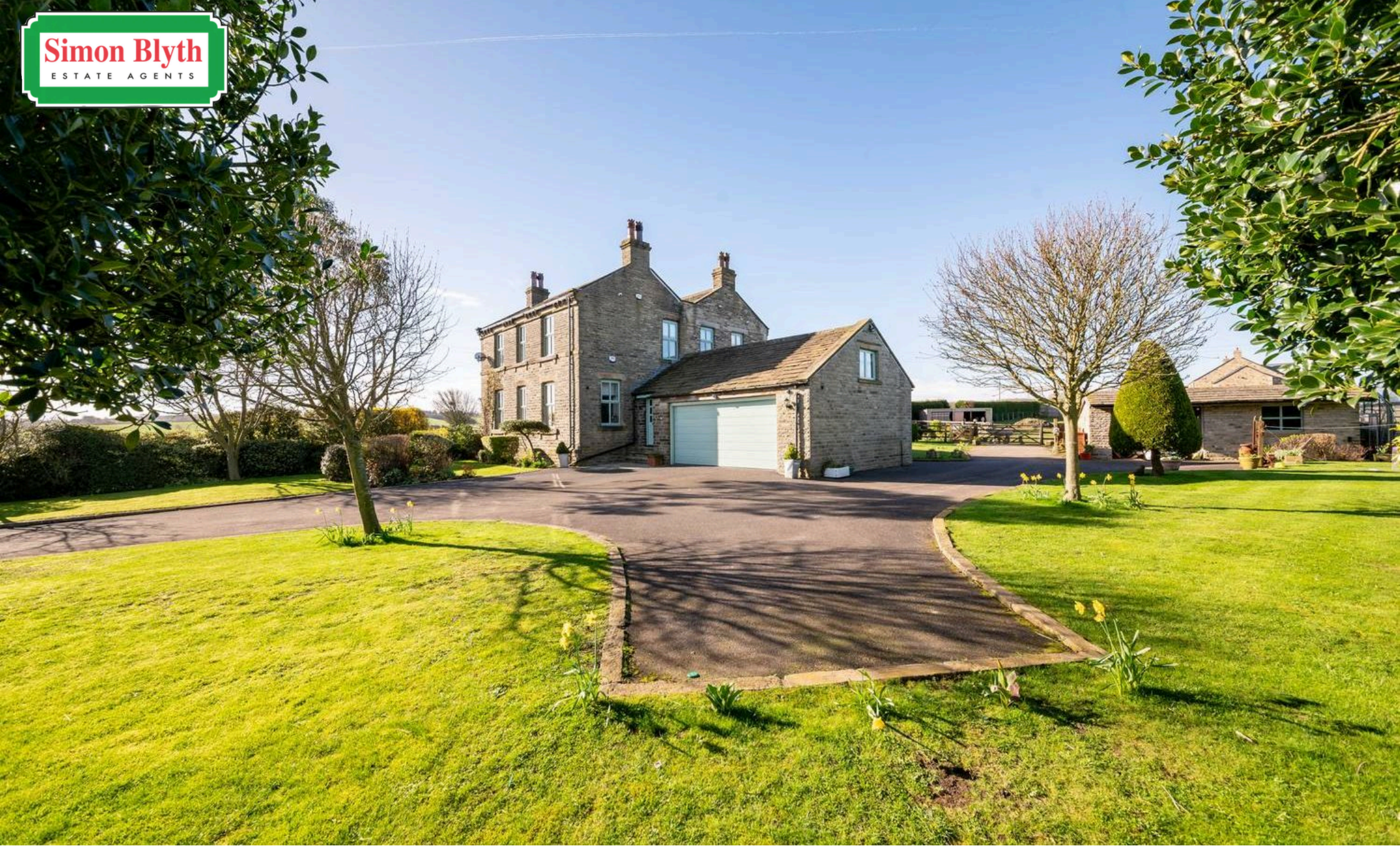
Reservoir House, Whitley Road, Whitley Whitley
