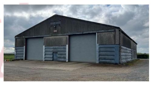
Dutch Barn, 18.46m x 7.72m, of steel frame construction, with corrugated tin walls and roof, soil floor. Lean to extension (18.46m x 7.74m) to the south, soil floor.
