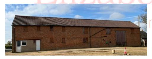
North Grain Store with electric shutter roller door and concrete floor. South Grain Store with manual sliding doors and wooden drying floor. Central drying tunnel, main air duct and laterals. A fan house is located on the north side of the building. 800 tonnes storage, 200 tonnes either side of central drying tunnel, each side. External measurement 18.29m x 27.43m.
