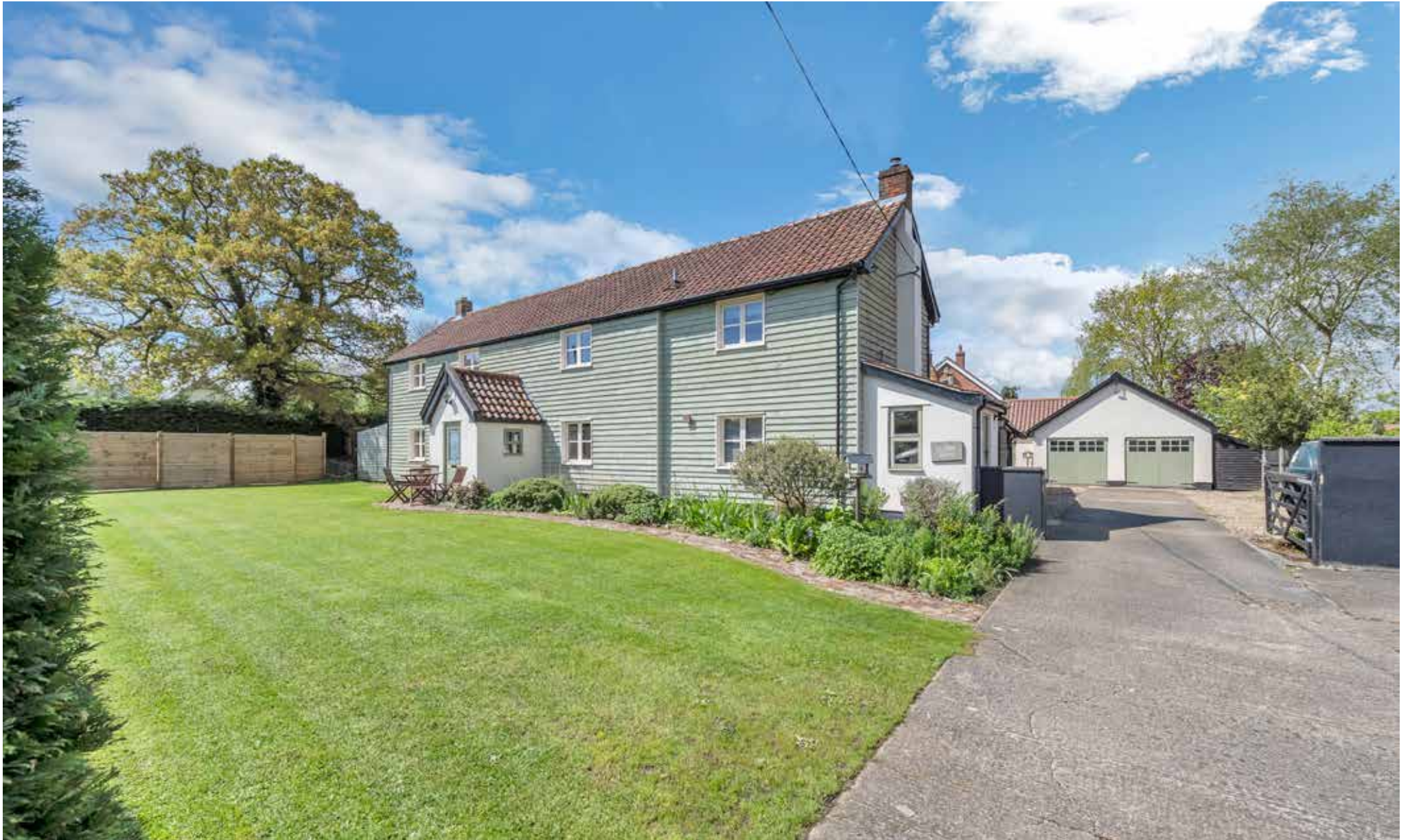
Clubbs House Denham Road | Hoxne | Suffolk | IP21 5DB
